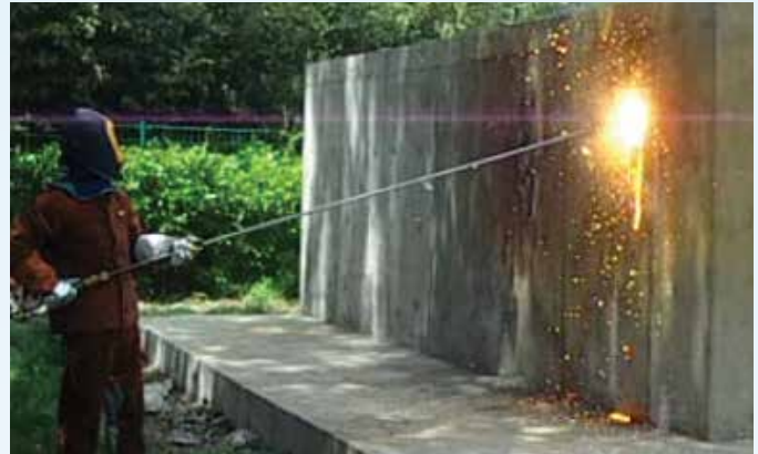
Thermic Lance at over 2500°C
